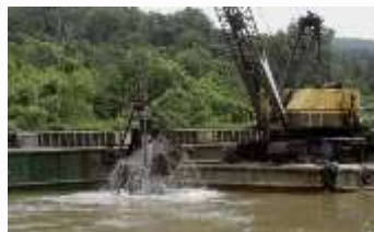
A dredger pulls sand out of Cambodia's Tatai River
